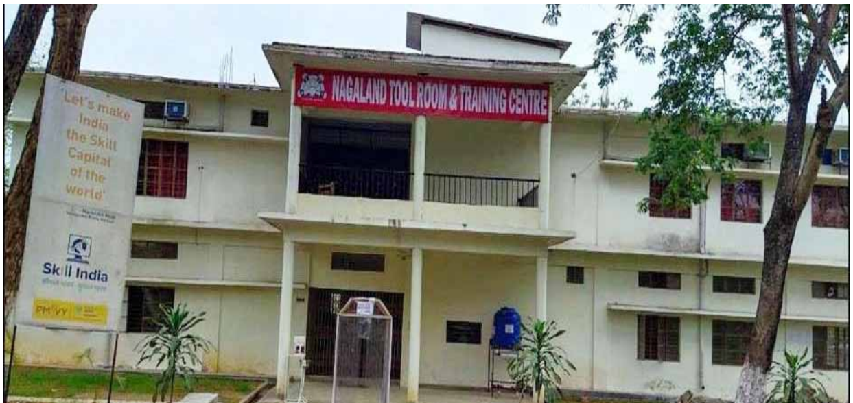
Front view of building NTTC, Dimapur
